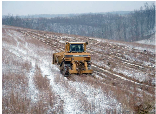
Figure 5. A standard single-shank ripper preparing a mine site for reforestation. The soil-ripping “tooth” being pulled by the dozer is intended to loosen soil material to a depth of 3 feet or more. The best results are achieved if this operation is performed in late summer and fall when the soil is dry.
