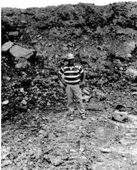
Figure 5. The 15-foot surcharge preloading fill at the Red Onion Prison site during surcharge removal. The excavation supervisor is standing on surcharged fill after partial surcharge removal with remaining surcharge material in the background.
