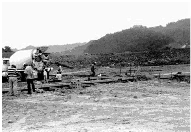
Figure 6. Pouring footings at the Red Onion Prison site after site stabilization. The surcharge fill is visible in the background of the photo.
