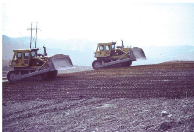
Figure 8. Typical grading and tracking-in operations for nonforest postmining land uses.
