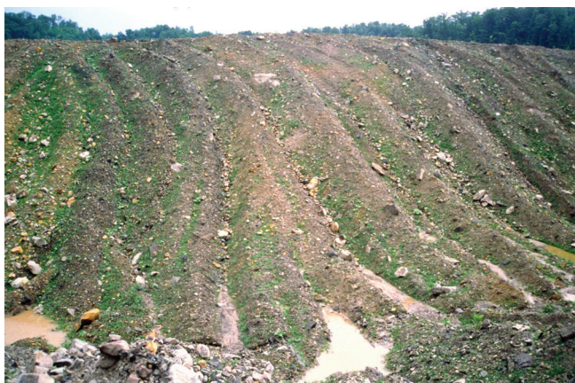
Figure 9. Example of uncompacted, roughly graded surface ideal for tree planting.
