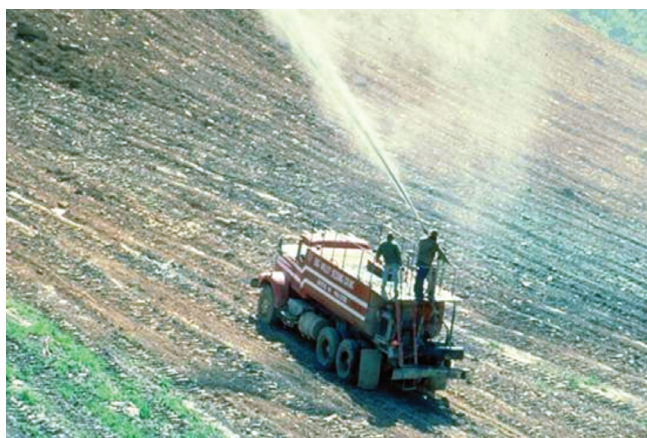
Figure 5. A hydroseeder applying seed in a fertilizer slurry while revegetating a surface coal mine.
